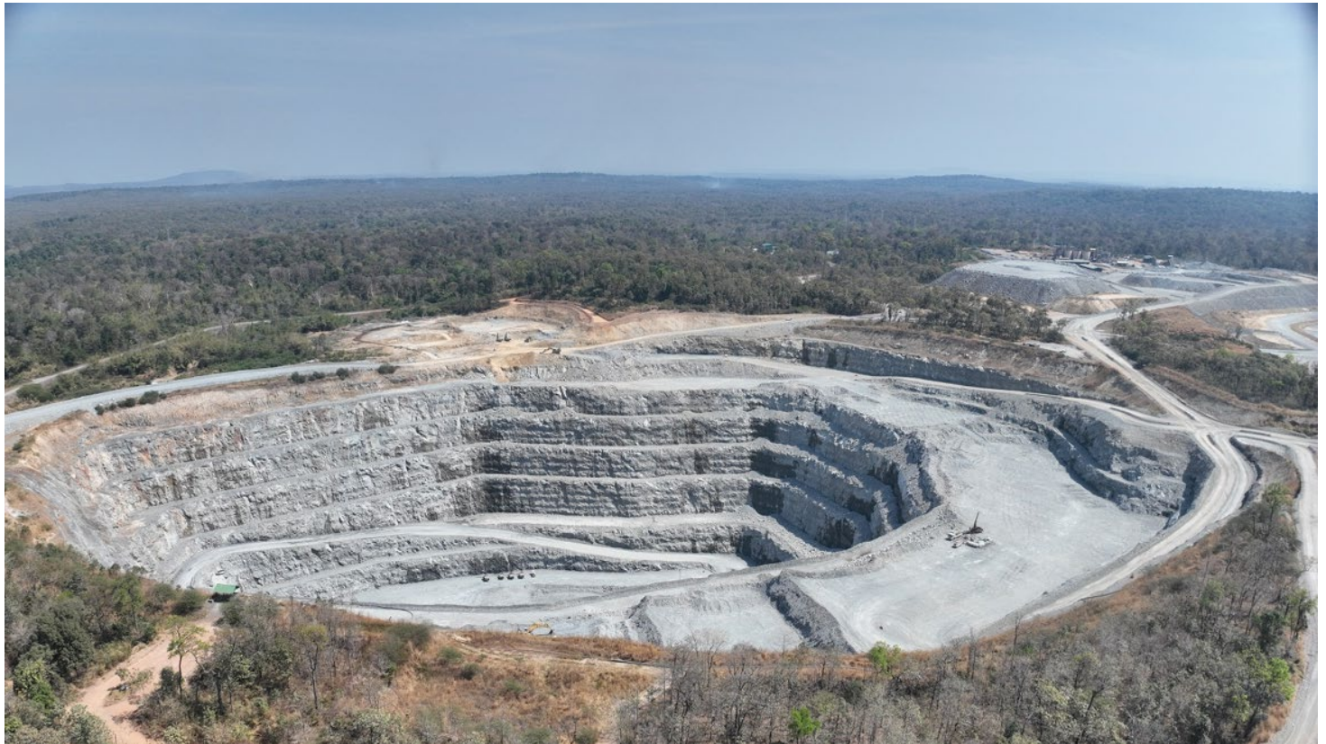
Figure 1 | Okvau Open Pit – January 2024
