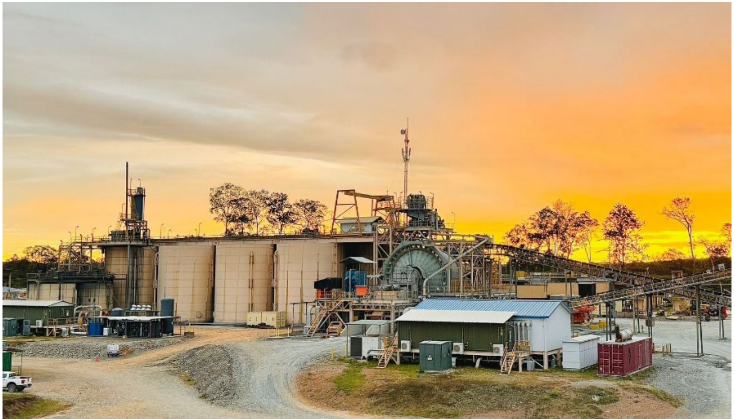
Figure 3 | Okvau Gold Mine Processing Plant
