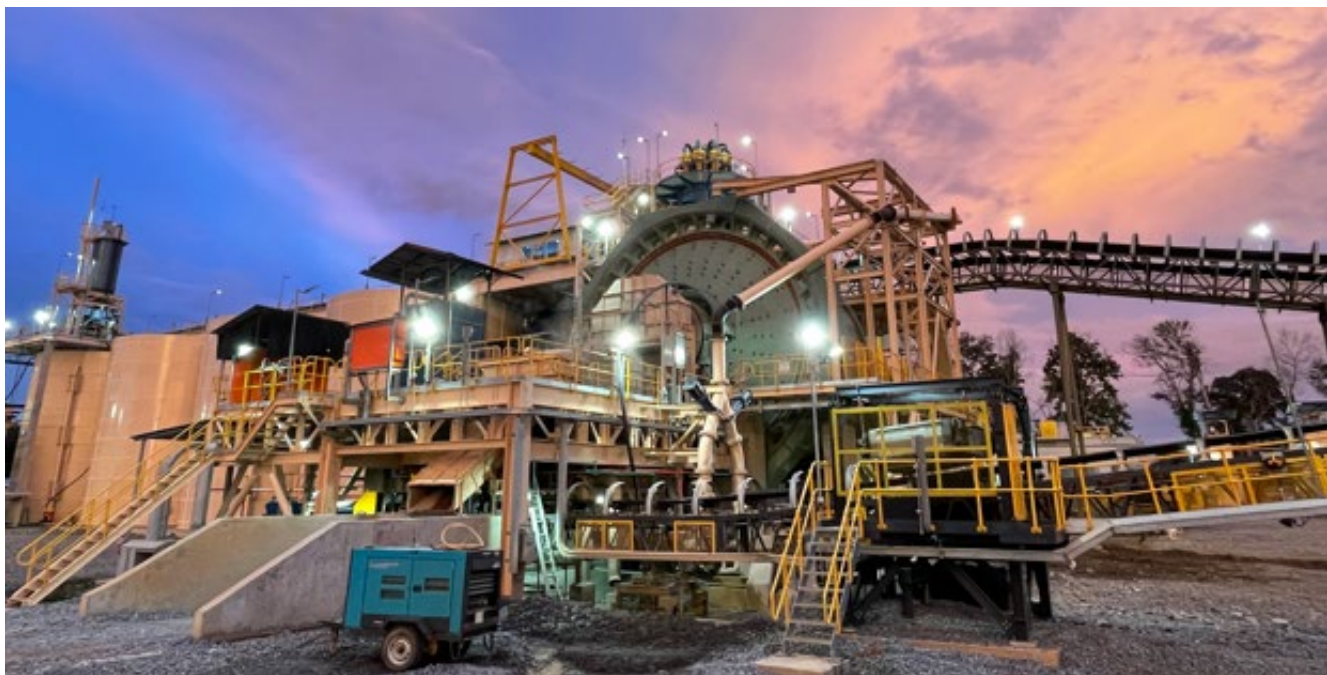
Figure 3 | Okvau Gold Mine Processing Plant
