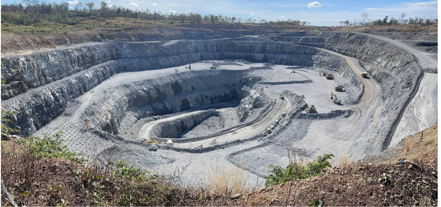
Figure 1 | Okvau Open Pit - January 2023
