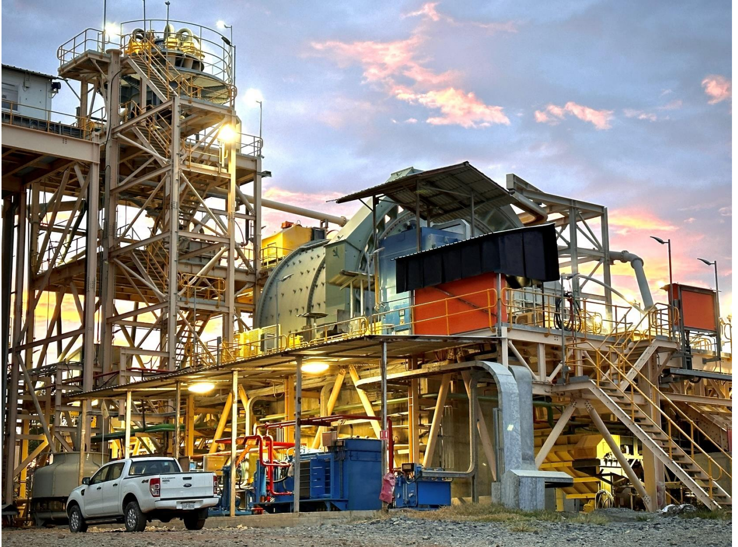
Figure 3 | Okvau Gold Mine Processing Plant - December 2022
