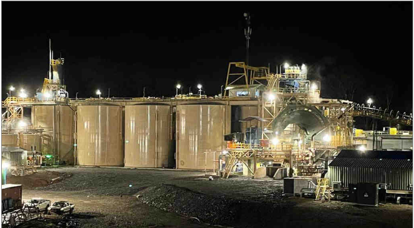
Figure 3 | Okvau Gold Mine Processing Plant
