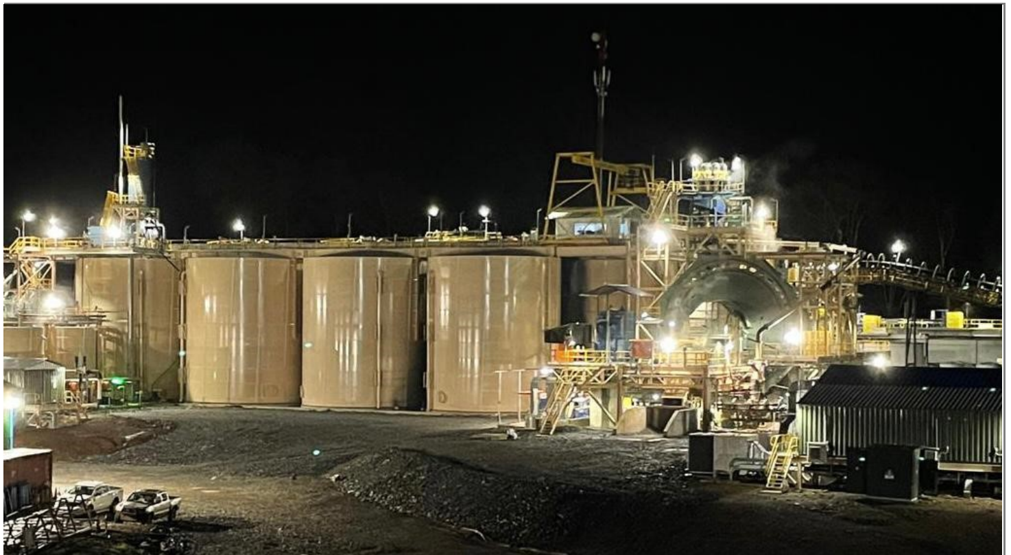
Figure 3 | Okvau Gold Mine Processing Plant
