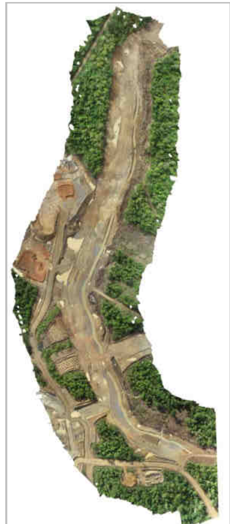
Figure 9 | Okvau Tailings Storage Facility (North Wall) - progressing on schedule
