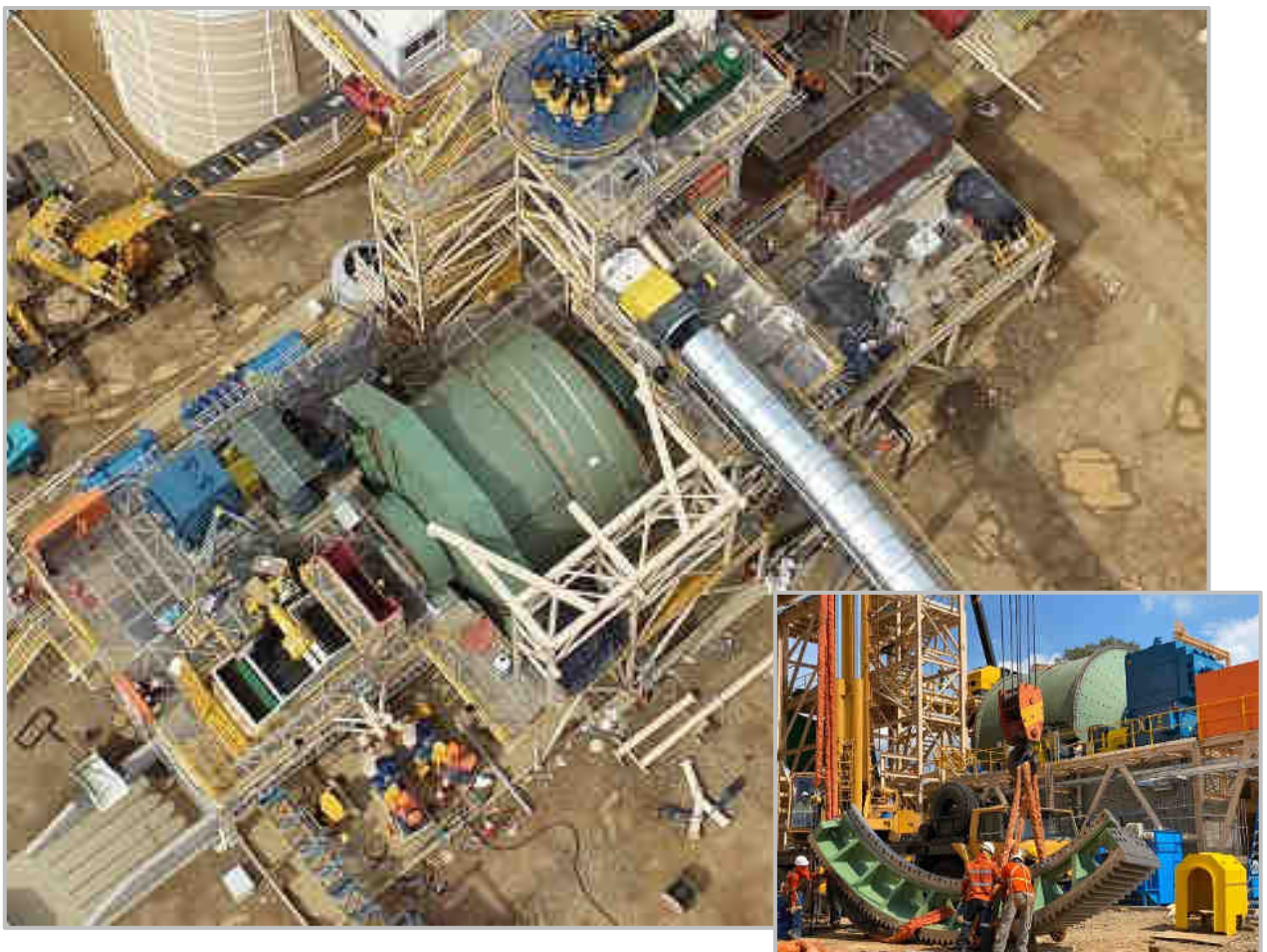
Figure 3 | SAG Mill installation nearing completion
