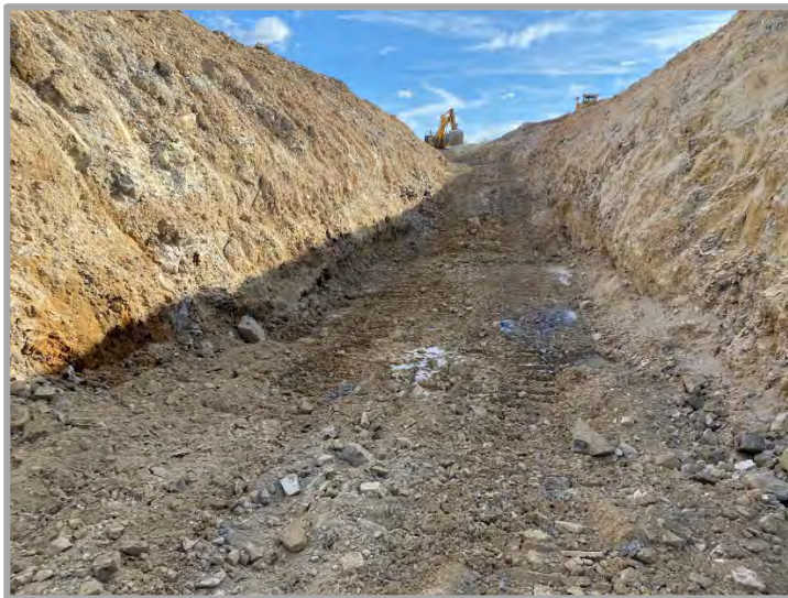
Figure Sixteen | Tailings Dam works & Keyway Excavation works
