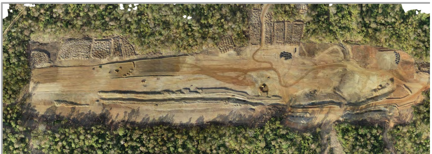
Figure Six | Tailings Dam Footprint Cleared, Topsoil stockpiled and Keyway cut
