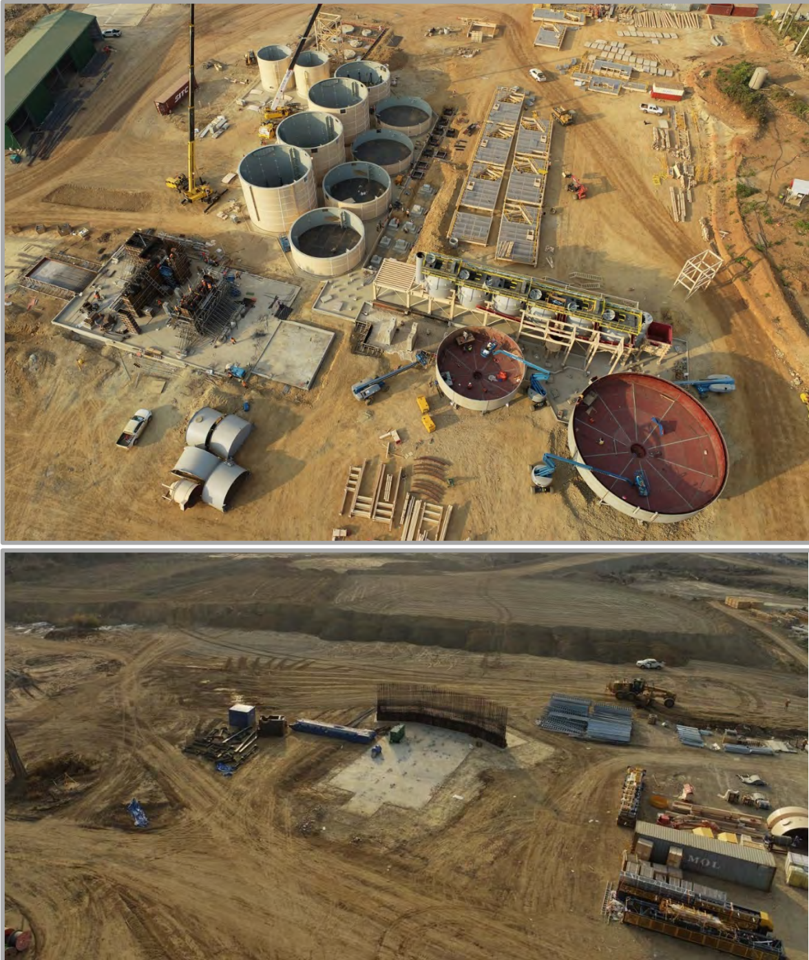
Figure Four | Plant Area-Tanks-Flotation-Mill Concrete-Crusher Concrete and ROM
