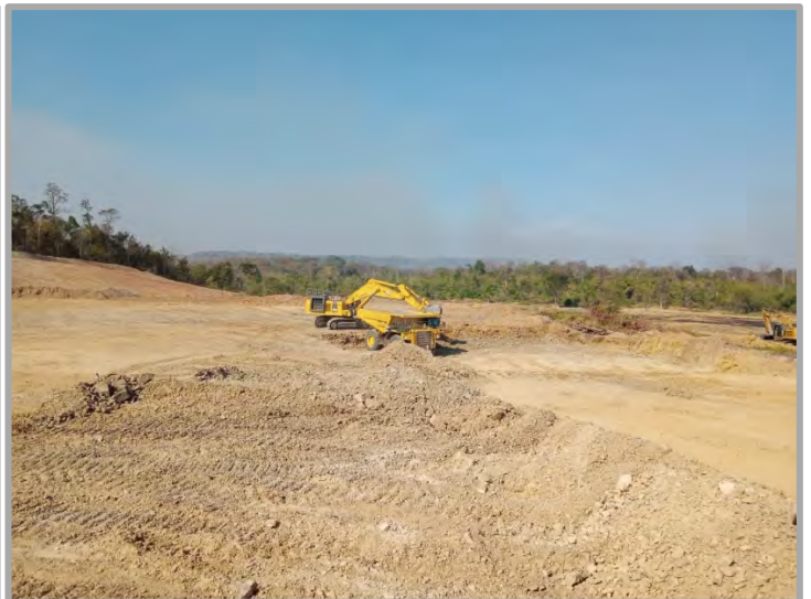
Figure Seventeen | Progress of Excavation works
