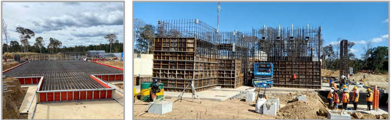
Figure Five | Primary Crusher Foundation Preparation
