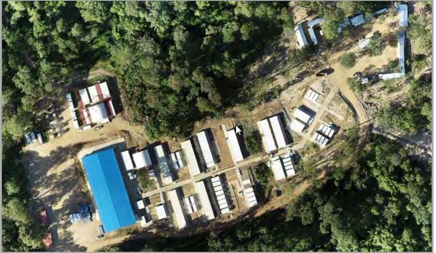
Figure Three | Okvau Accommodation Village Overview
