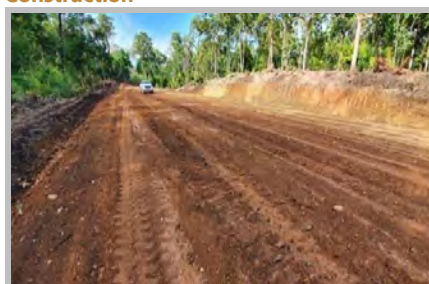
Figure 24 | Haul and Site Access Road Construction
