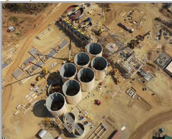
Figure 18 | CIL Tanks
