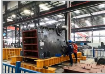
Figure 11 | Trial Assembly of Primary Jaw Crusher
