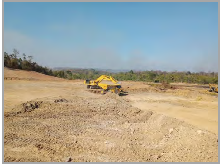
Figure 22 | Progress of Excavation works
