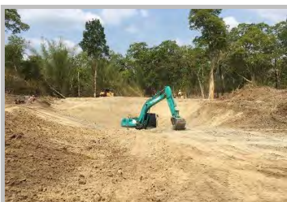
Figure 23 | Process Plant Sediment Pond
