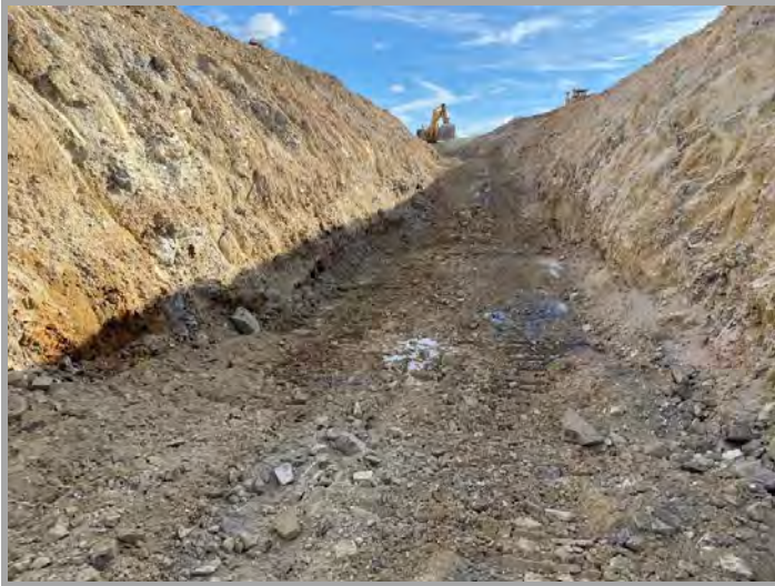
Figure 21 | Tailings Dam - Keyway Excavation works
