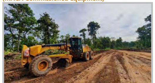
Figure 25 | Contractor Yard Clearing (MACA Commissioned Equipment)
