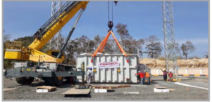
Figure 27 | Installation of Transformer
