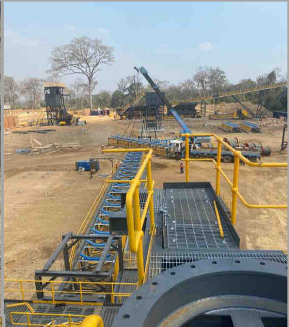
Primary Crusher Installed
