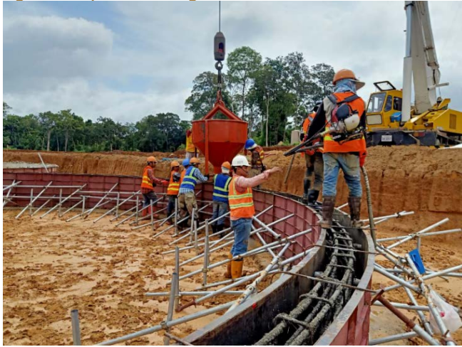
Figure Nine | CIL Tank Ring Beams
