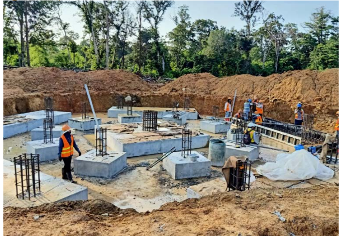
Figure Ten | Float Cell Foundation
