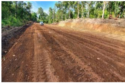
Figure Twelve | Haul and Site Access Road Construction
