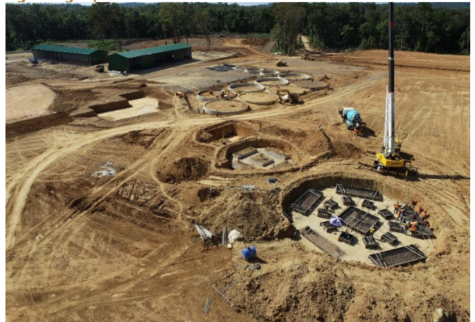
Figure Eight | Process Plant Civils
