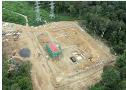
Figure Two | Substation Civil Works Aerial view
