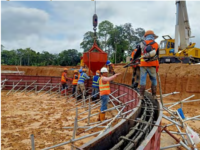
Figure Fourteen | CIL Tank Ring beams
