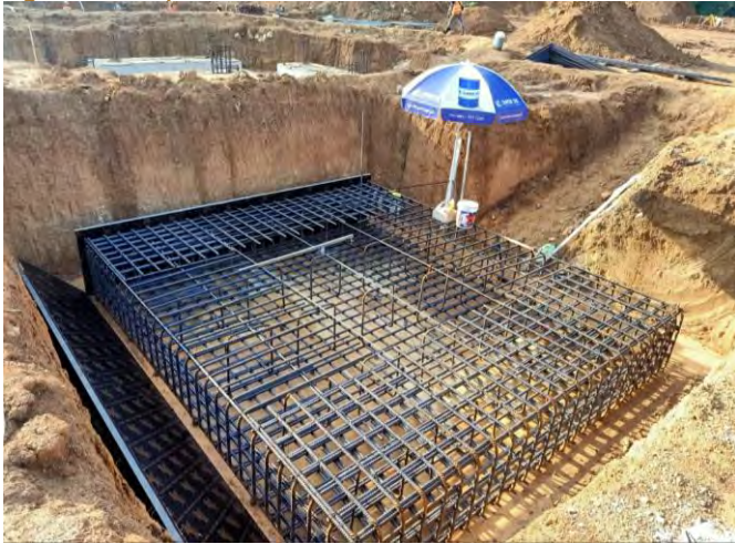
Figure Twelve | HIG Mill Foundation
