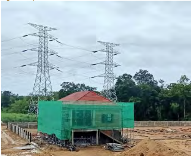
Figure Six | Substation Civil Works
