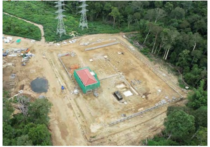
Figure Seven | Substation Civil Works Aerial view
