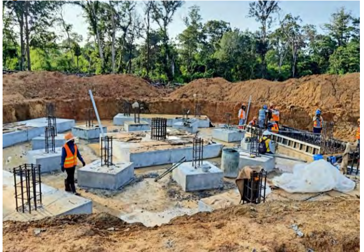
Figure Thirteen | Float Cell Foundation
