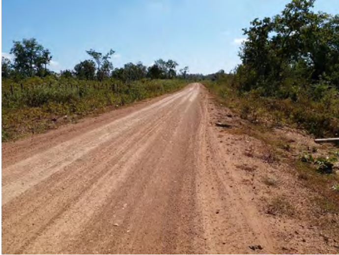
Figure Four | Okvau Access Road
