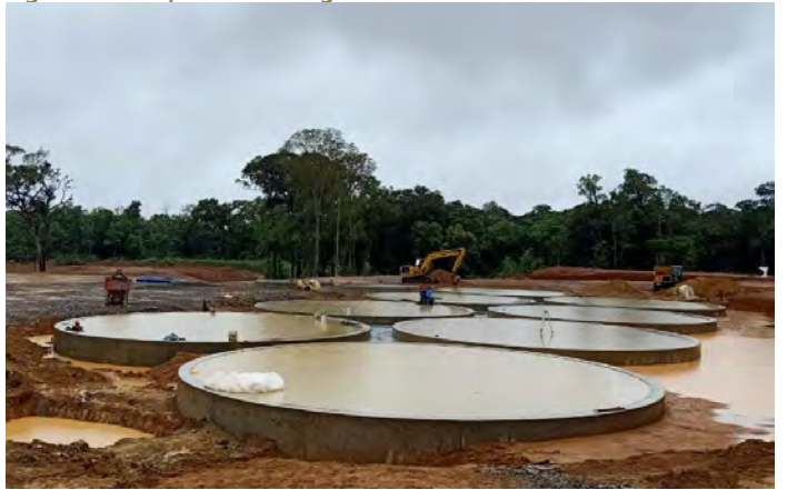
Figure Fifteen | CIL Tank Ring beams
