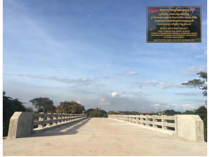
Figure Five | Prek Te River Bridge
