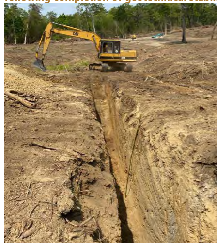
Figure Seventeen | Plant site cleared and topsoil pushed up following completion of geotechnical stability assessment
