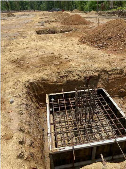
Figure 5 | Substation Footings
