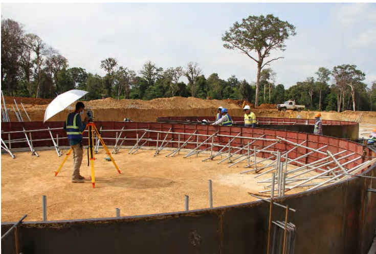
Figure 4 | CIL Tank Ring beams
