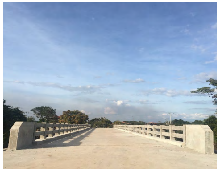
Figure 4 | Prek Te River Bridge
