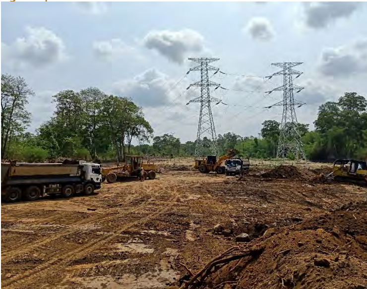
Figure 5 | Substation Civil Works
