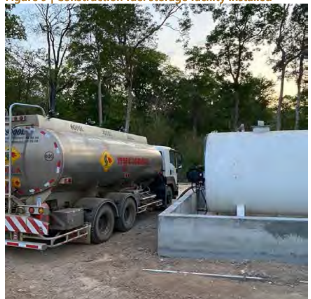
Figure 9 | Construction fuel storage facility installed
