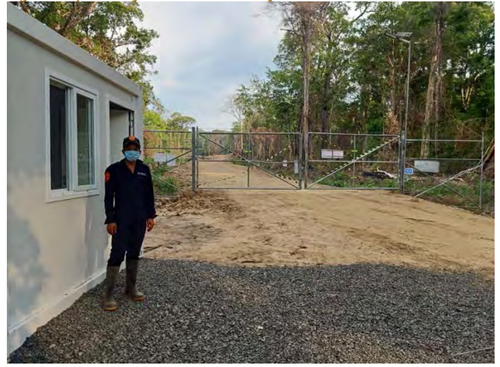
Figure 23 | Security Gate at Okvau Project
