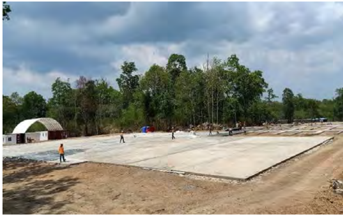
Figure 7 | Village Construction Works
