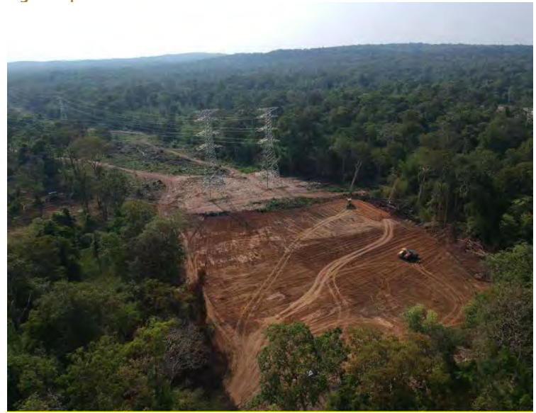
Figure 6 | Substation Civil Works Aerial view
