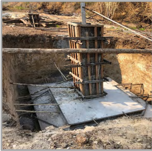
❑ Tower Footings on Okvau PDA.
