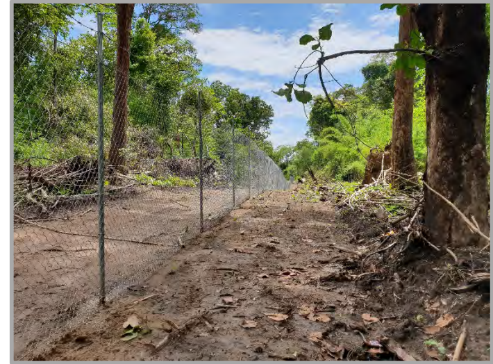
❑ Okvau PDA Fencing Complete.
