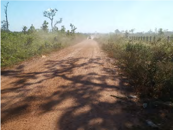
Figure 8 | Okvau Access Road, materially complete
