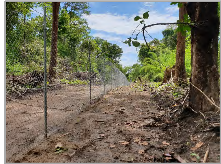
❑ Okvau PDA Fencing Complete.
